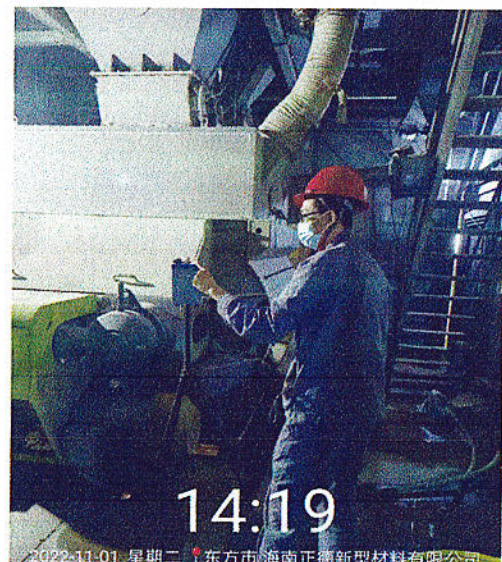
搅拌机粉尘检测
